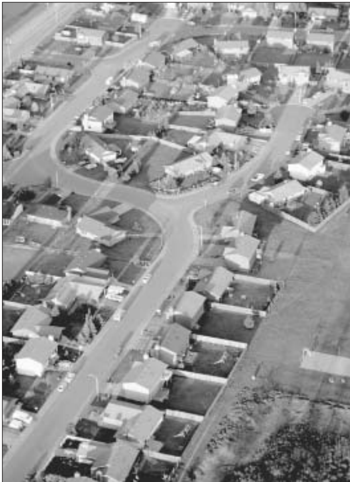
Narrow roads and smaller fire trucks would be the wisest choice, in order to handle fires as well as decrease the number of traffic accidents and fatalities.
